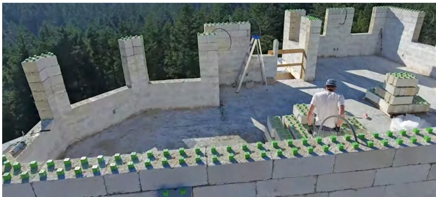
This video still shows the construction of a Vancouver Island home built with Just BioFiber’s modular blocks. photo: justbiofiber.ca
